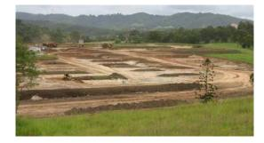
The need for compensatory earthworks for flood mitigation requiring the placement of bio-retention basins above major storm levels presented technical challenges for piped stormwater conveyance systems.
