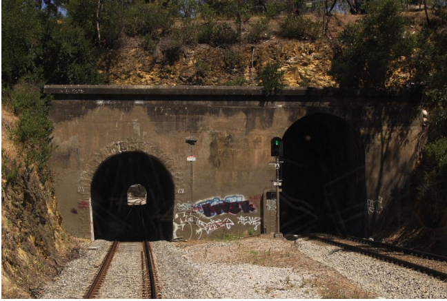
Approaching the Eden Hills tunnels
