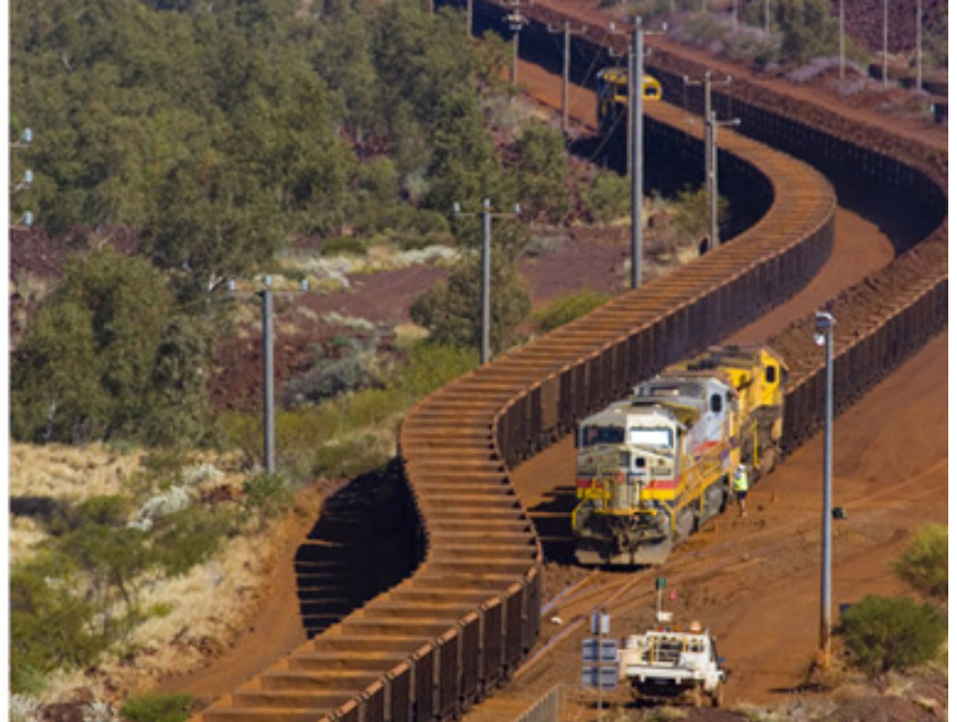
Iron ore rail facilities
